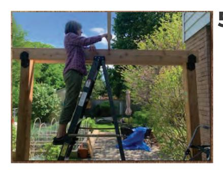
Once you have your posts and beams up and in position, take your first rafter, and place in the centre of the beams, again with each rafter overhanging the outside beam by approximately 12". You will fasten the rafters to the beams using the APA21 Ornamental Angle (rafter tie clips) using the 1-1/2" black screws. We supply enough rafter tie clips to fasten the rafters to the beams on the outside, and inside beam so you will see the black accents inside and outside of the Pergola.
