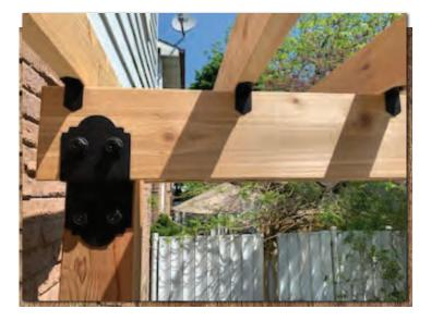
6. After installing the centre rafter, continue to place the remaining rafters 12" apart on centre, they should end approximately 12" away from the end of your beams.
